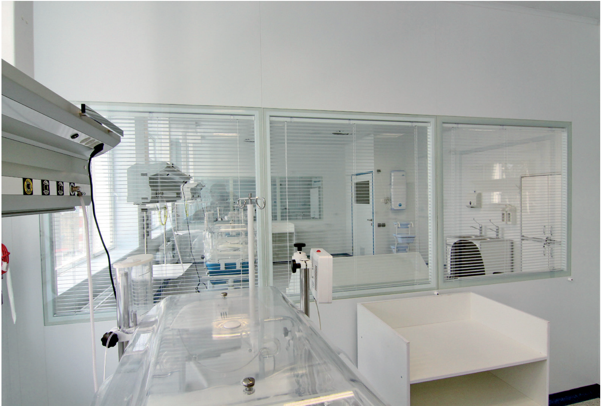
Building in 4 operating theatres | Regional perinatal centre | Voronezh, Russian Federation | 2011
