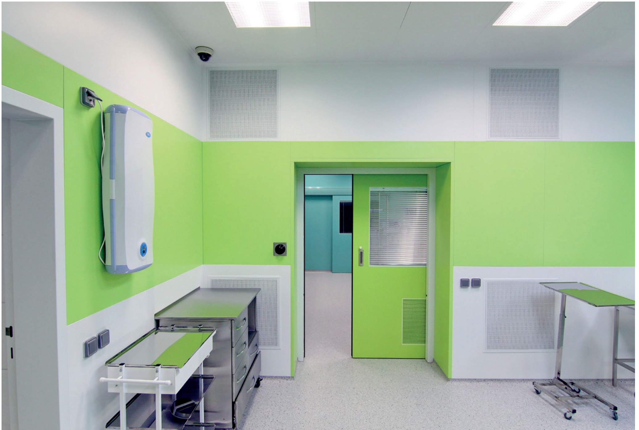
Building in 4 operating theatres | Regional perinatal centre | Voronyezh, Russian Federation | 2011
