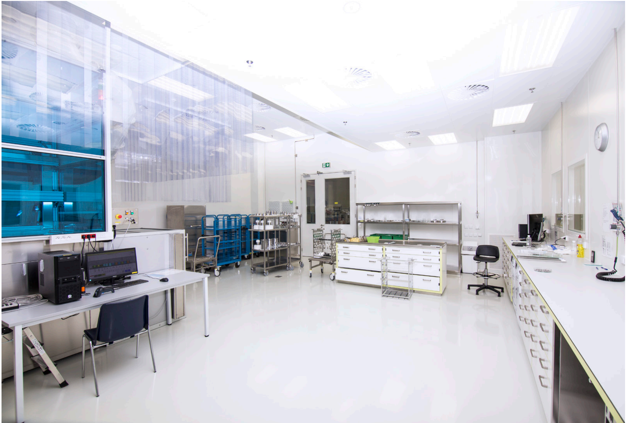
New Operations Facility CTPark Brno | FEI Czech Republic s.r.o. | Brno, Czech Republic | 2014
