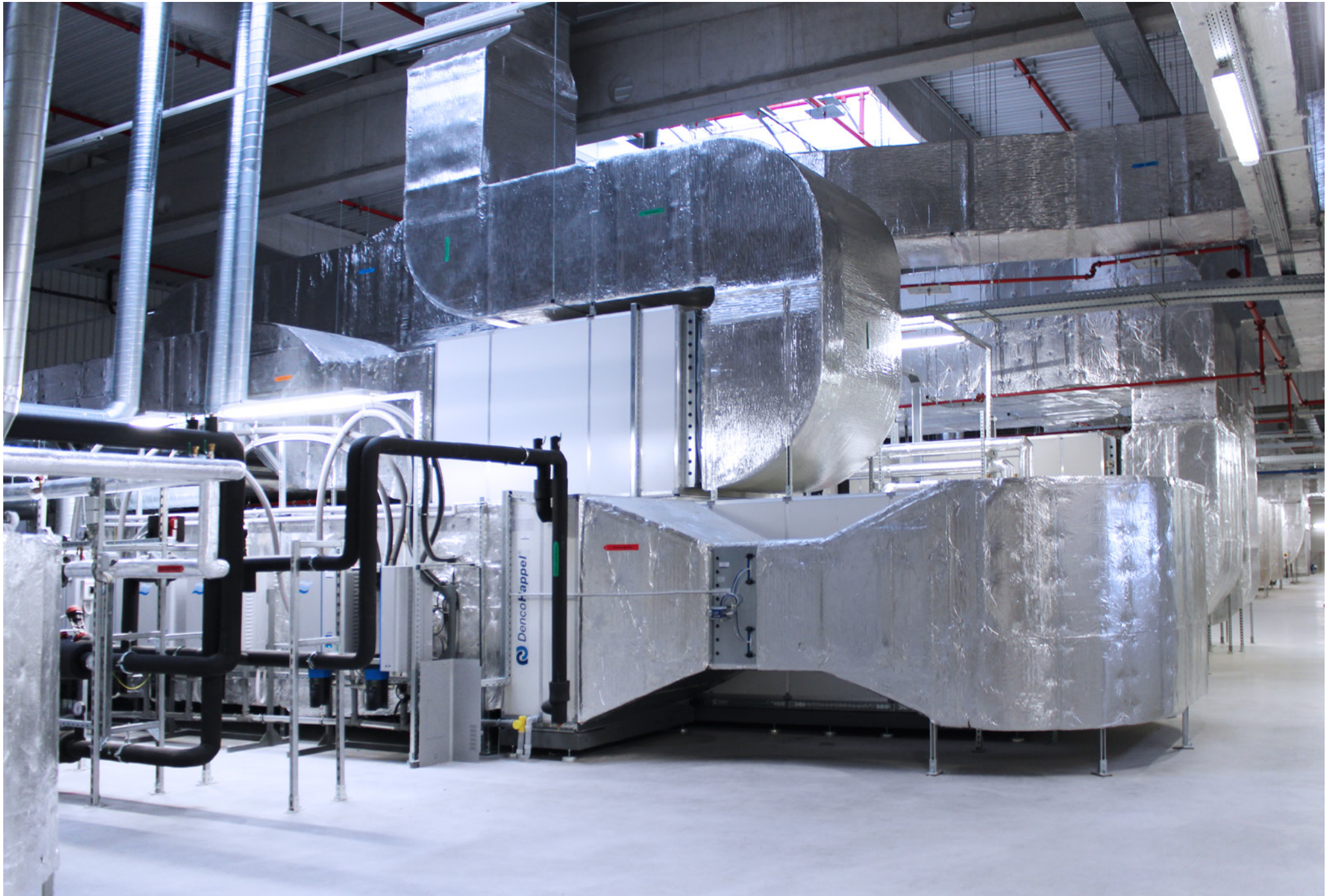
D2.3 Laboratory Building; Thermo Fisher Scientific Brno s.r.o.; Brno; Czech Republic; 2019
